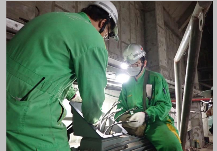
Wind turbine motor replacement
