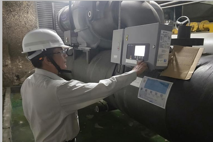
Chiller equipment maintenance
